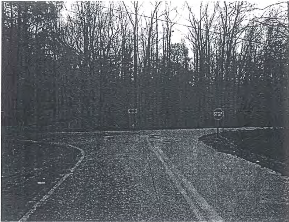
Fickling Hill Road (Looking East) at Brownswood
